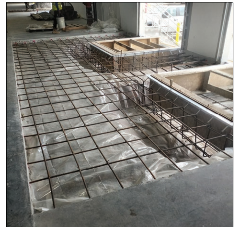
Proper reinforcement ensures strength, durability, and long-term performance.
