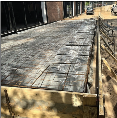
Rebar reinforcement for a commercial business development's new sidewalk.
